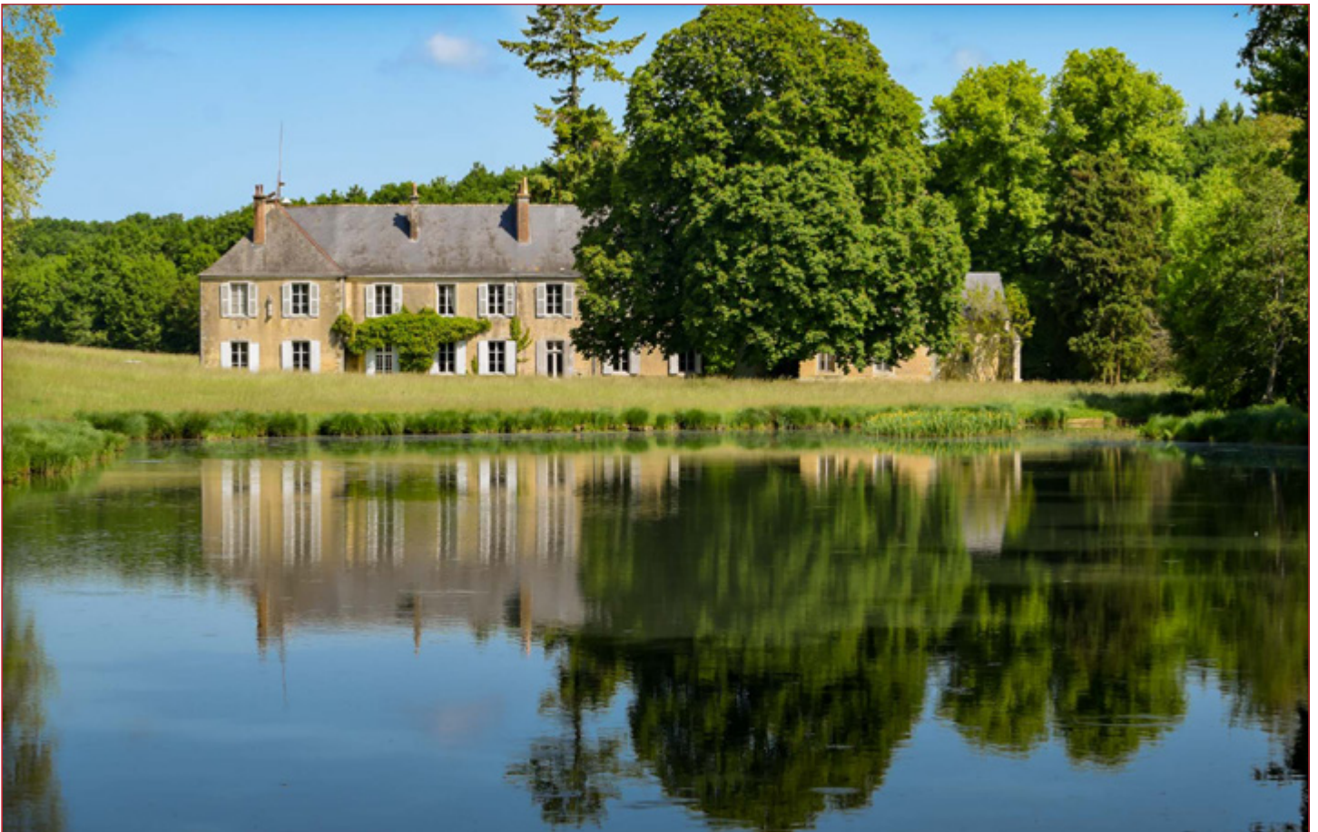
THE MAIN HOUSE (FOR MORE INFORMATION VISIT BONNEVAUXWCCM.ORG )
